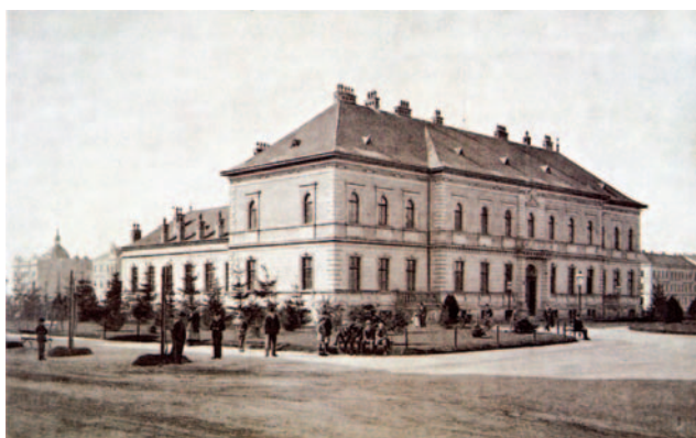
Fig. 5: The university chemical department building at the Academy Square (today's Stroussmayer Square 14), where the Pharmacognosy Institute was initially located. Photo around 1895.
