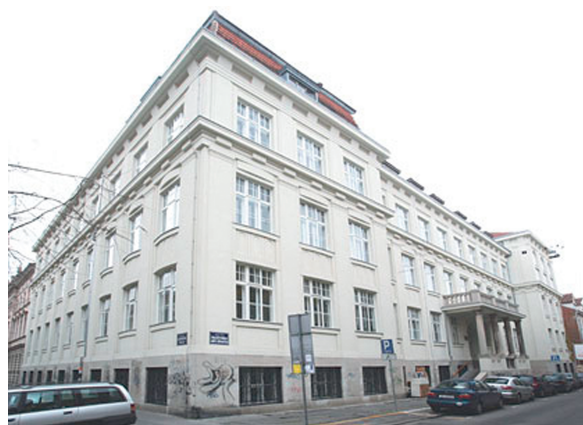
Fig. 6: The central building of the Faculty of Pharmacy and Biochemistry of the University of Zagreb, situated at No. 1 of Kovačić Street.
