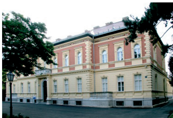
Fig. 5: The former building of the Chemistry Institute at No. 14 of Strossmayer Square in Zagreb. Today it houses the CASA Library.
